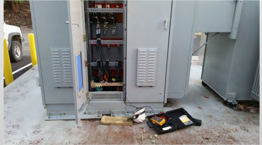
Fire Station Electrical Upgrade
